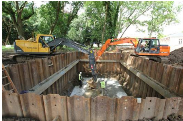
2. Excavation for 22 000 litre tanks
